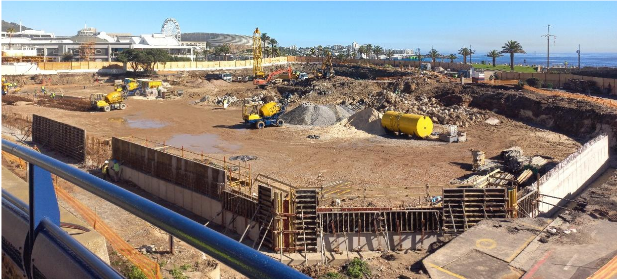
Figure 2. Construction of another development occurring south of the proposed site. Parcel P is located to the right of the construction area (not fully visible), while Parcels O and a1 and a2 are visible in the distance near the grassed area and palm trees.
