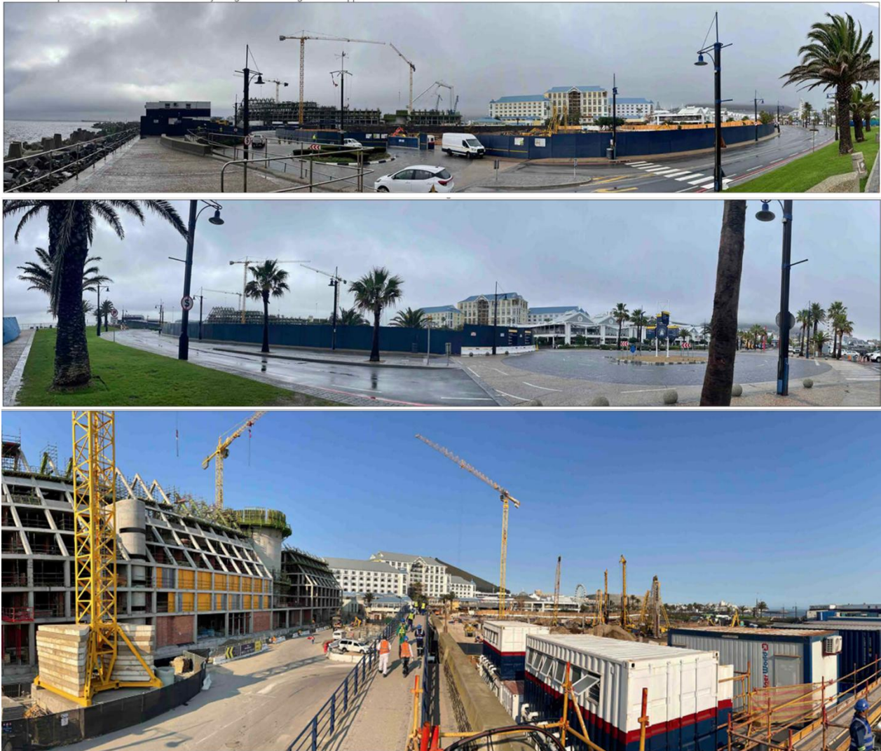
Figure 30. Top: View from the circle at the roadway to the Table Bay Hotel. Although Signal Hill is covered in cloud in this image, the “frame” set up by the Quay 7 hotel building (under construction) and the Table Bay Hotel is evident. The promenade-like qualities of the walkway along the coastal edge are also apparent. Middle: View from the elevated coastal walkway in front of the Table Bay Hotel. Although Signal Hill is covered in cloud in this image, the “frame” to the subject site that is set up by the Quay 7 hotel building (under construction) and the Table Bay Hotel is evident. The promenade-like qualities of the walkway along the coastal edge are also apparent. Bottom: View from the Breakwater Wall looking over the site (with a basement being constructed). Signal Hill, the Cape Wheel and Cape Town Stadium are visible, as is Granger Bay. To the east, the Quay 7 Hotel blocks views towards Victoria Basin and Table Mountain.
