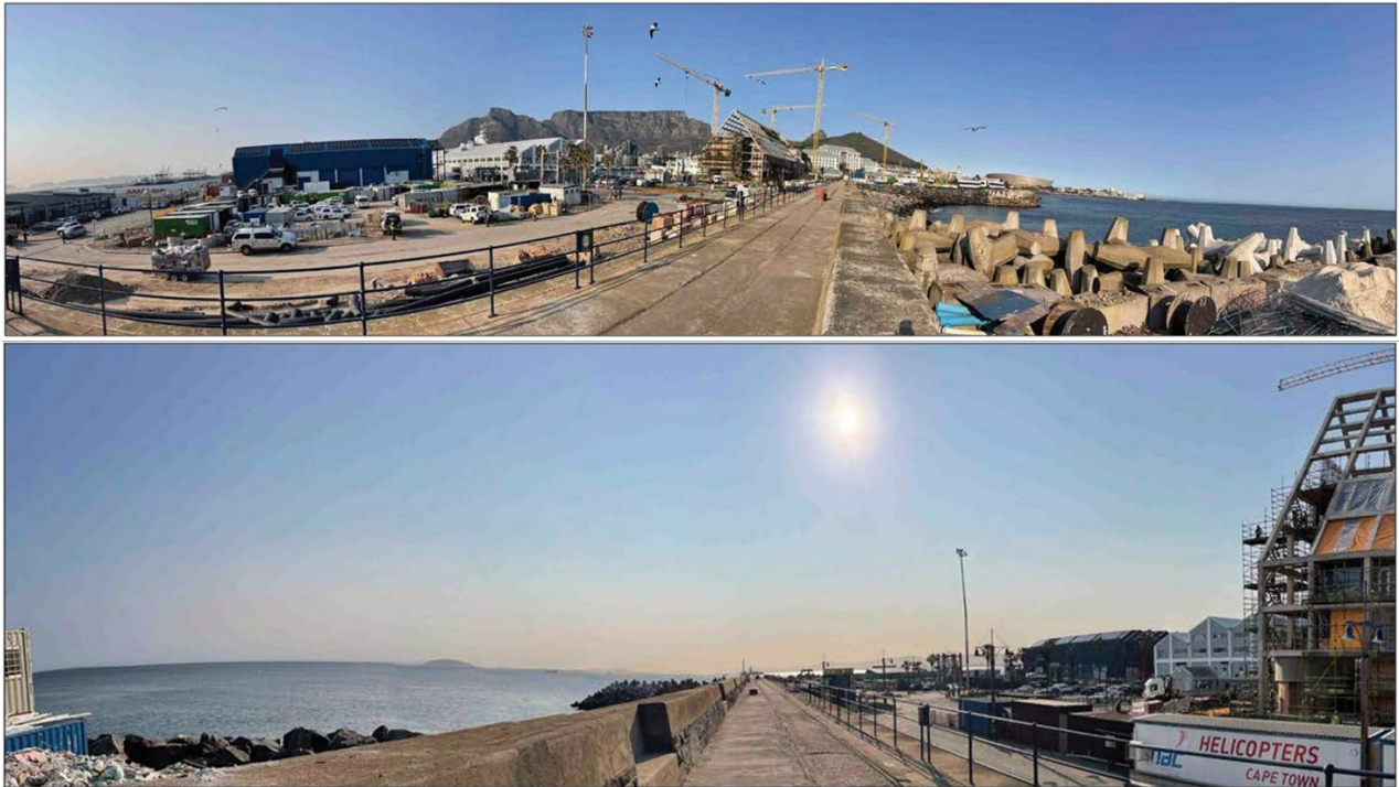
Figure 28. Top: Views attained from the Breakwater allow for strong visual connections between Table Bay and the Mountain Range - key to Cape Town's sense of place. Bottom: Views from the Breakwater Wall towards Table Bay allow for a sense of placement and orientation within the bay.
