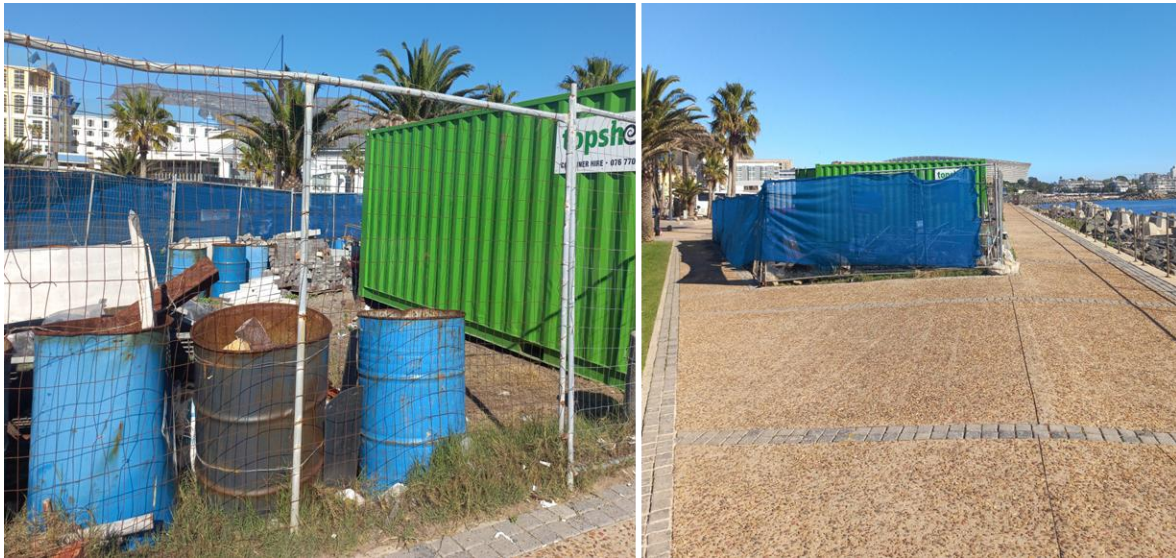
Figure 5. Containers and construction material temporarily present in the area, partially overlapping with and situated in front of proposed Parcel O.
