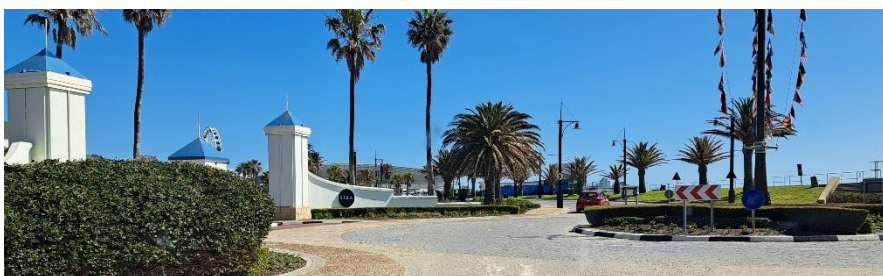
Figure 17: Breakwater Boulevard north-west bound, site ahead, no visibility of the sea
