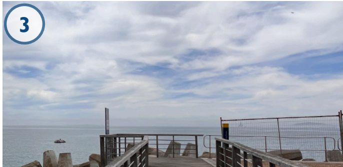
EXISTING CONDITIONS: PEDESTRIAN VIEWS TOWARDS ROBBEN ISLAND AND BLOUBERG ARE ALONG THE ELEVATED BOARD WALK
