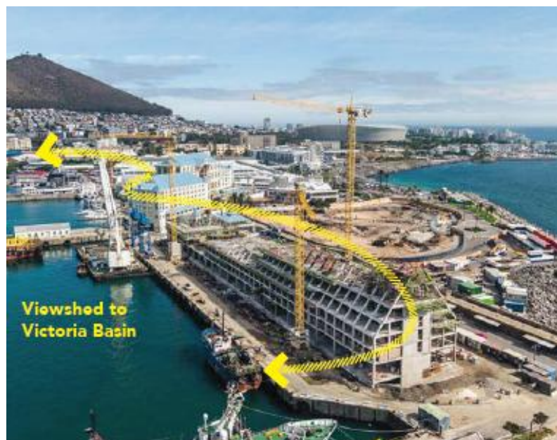
Figure 88B: Drone view of the Quay 7 building under construction clearly show that the structure creates a visual “viewshed” between the Victoria Basin and the site. (Sources: https://hodari.co.za/project/hotel-and-luxury-residence-development-2/ and GVK-Siya Zama).
