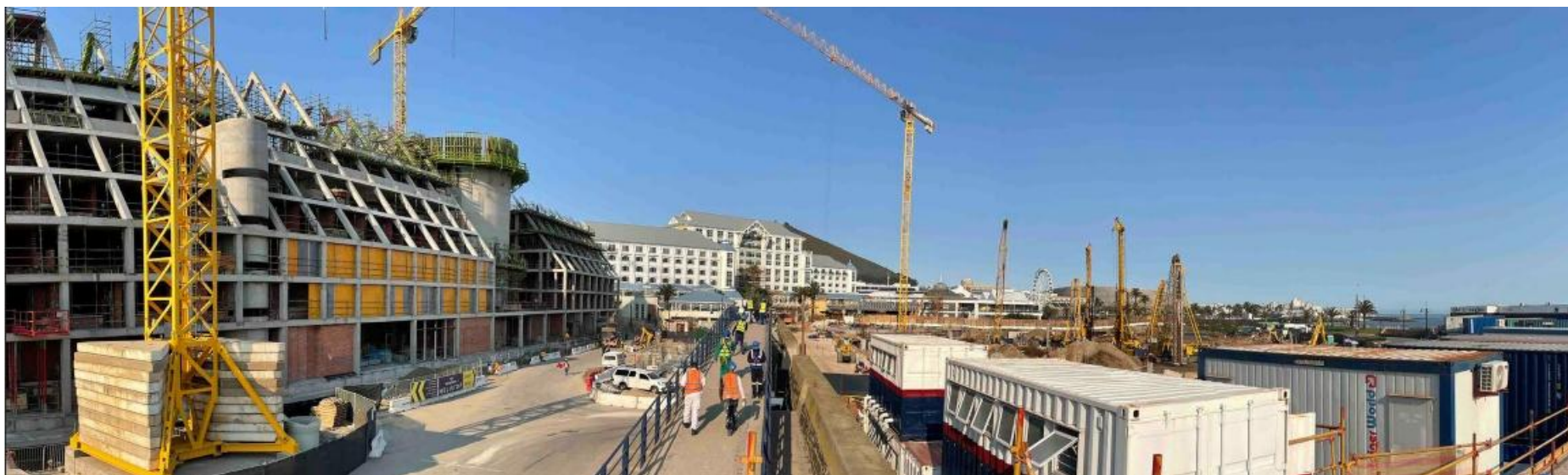
Figure 54.21G: View from the Breakwater Wall looking over the site (with a basement being constructed). Signal Hill, the Cape Wheel and Cape Town Stadium are visible, as is Granger Bay. To the east, the Quay 7 Hotel blocks views towards Victoria Basin and Table Mountain.
