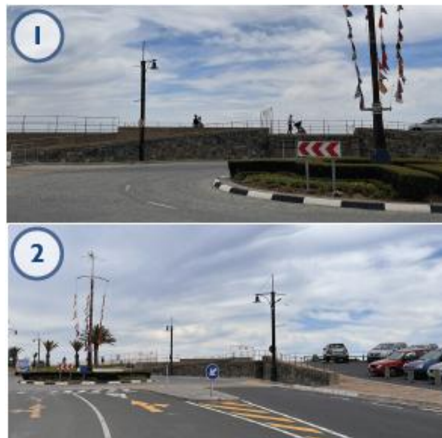
Figure 81: Existing conditions from Breakwater Boulevard toward the boardwalk (V&amp;AW).
