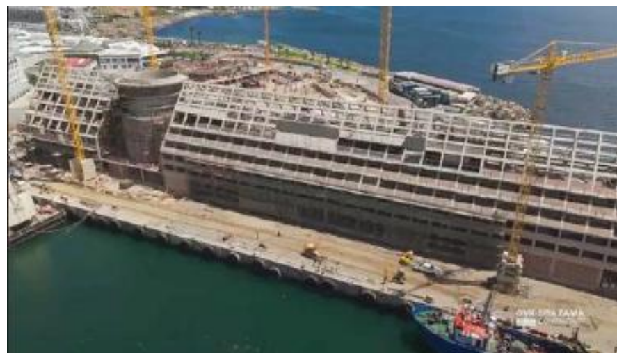
Figure 88C: Drone views of the Quay 7 building under construction clearly show that the structure creates a visual “viewshed” between the Victoria Basin and the site. (Sources: https://hodari.co.za/project/hotel-and-luxury-residence-development-2/ and GVK-Siya Zama).
