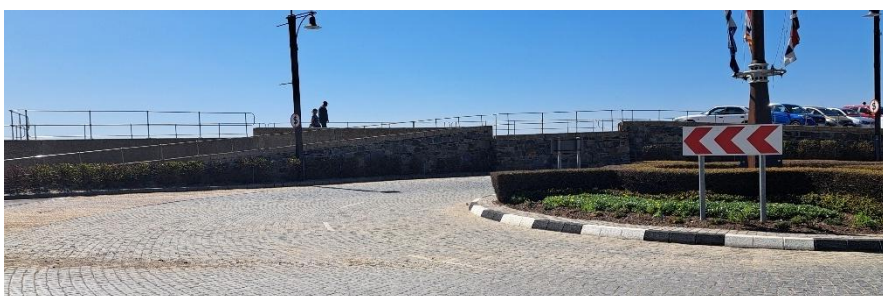
Figure 18: Breakwater Boulevard looking north, site and elevated coastal walkway ahead.
