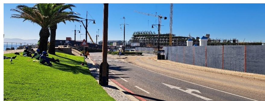
Figure 14: Breakwater Boulevard eastbound, site left and front. Quay 7 building in the background.
