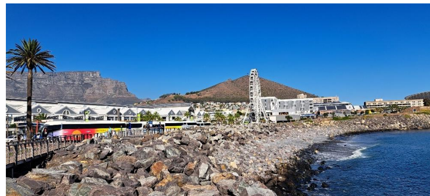
Figure 25: From the coastal walkway on site looking south west
