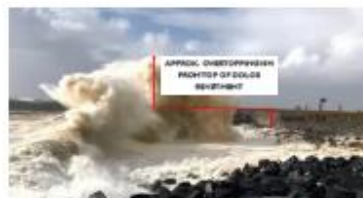
STORM CONDITIONS ERODING THE EXISTING COASTLINE DUE TO THE FORCE OF WAVES AND OVER-TOPPING
