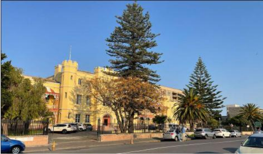
Figure 55.22E: Somerset Hospital is a stately landmark and a major organising townscape element for the precinct.
