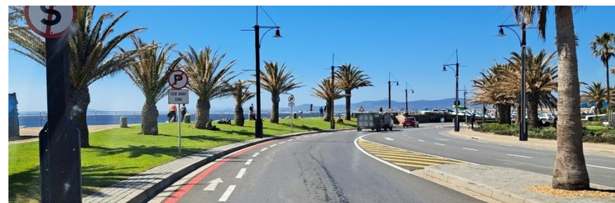
Figure 13: Breakwater Boulevard eastbound, site left
