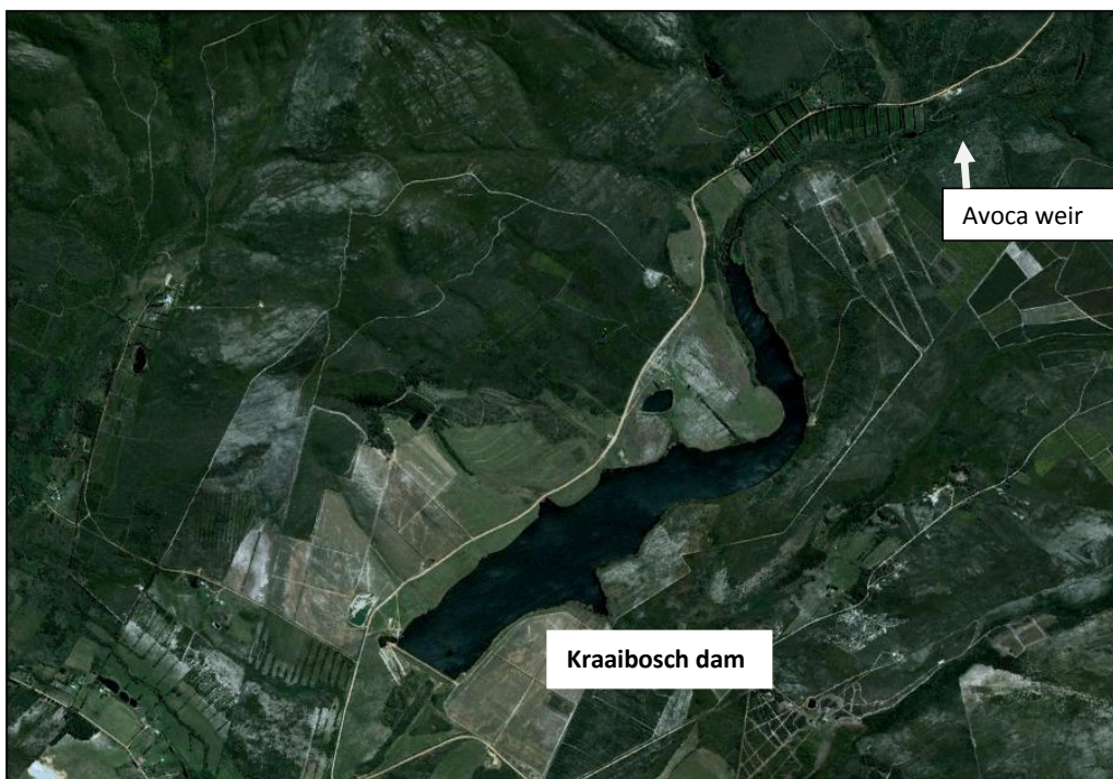
Figure 3.6. Kraaibosch Dam (Source: Google Earth)
