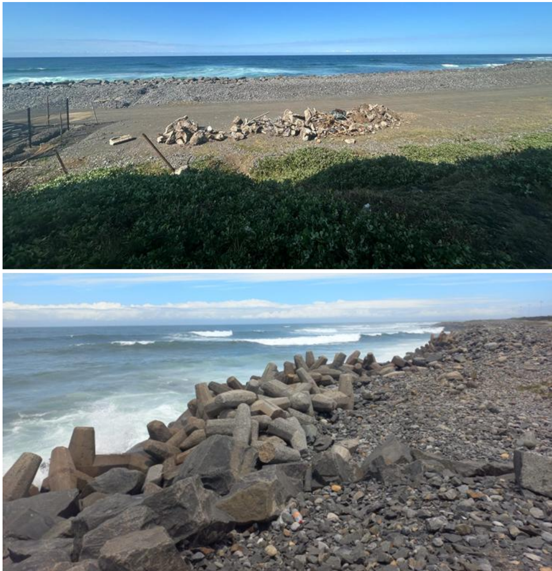
Figure 3.12. The outfall pipeline will cross the service road (visible in the top image) towards the breakwater and ocean. It will then traverse the breakwater, which comprises rock and dolosse (visible in the bottom image), and terminate at the outer edge of the dolosse, discharging into the ocean.
