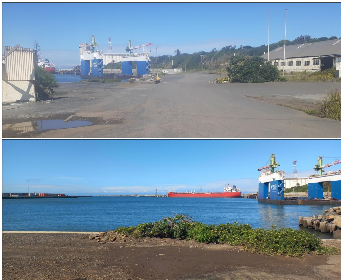
Figure 3.10. Views of the proposed estuarine intake and pumpstation site. Top: The proposed pumpstation would be situated in the centre-left of the pane, whereas the municipal substation is located just beyond the grey-roofed building to the right of the screen. Bottom: The proposed intake pipeline will protrude into the estuarine waters to the centre-right of the pane
