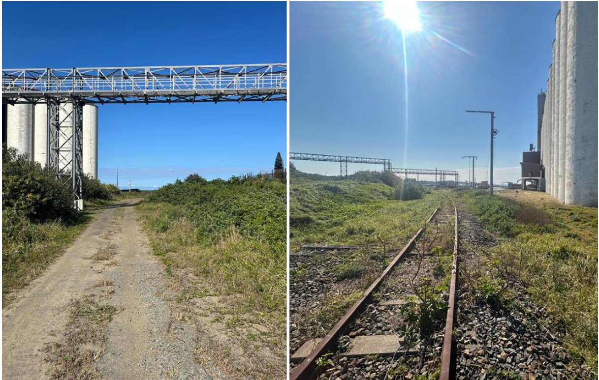
Figure 3.11. The pipeline will largely follow existing roads and railway lines within already disturbed and modified areas. The silos are visible on the right-hand side of the right photograph.
