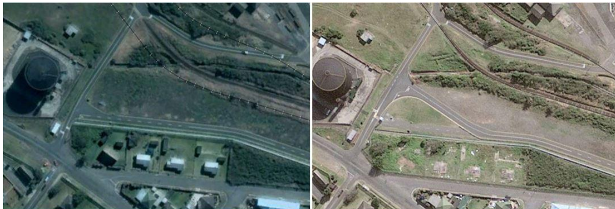
Figure 12: Consecutive Google Earth satellite images dated August 2004 (left) and August 2009 (right) showing the four houses on the proposed PV site, pre- and post-demolition (Source: Google earth).
